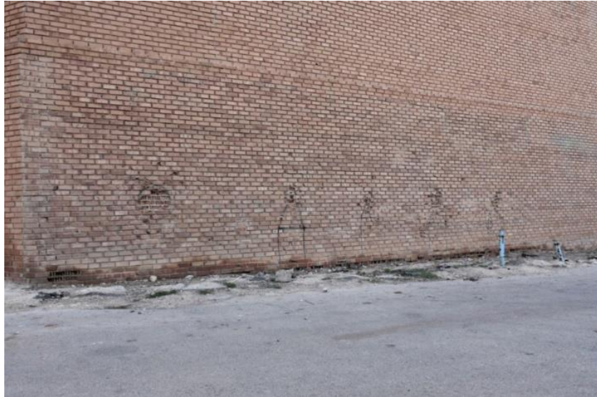
A picture showing the effects of the (Ashbal al-Khilafa) training on firing on the newly restored retaining wall in the western part of the walls of The Citadel of Ja'bar
