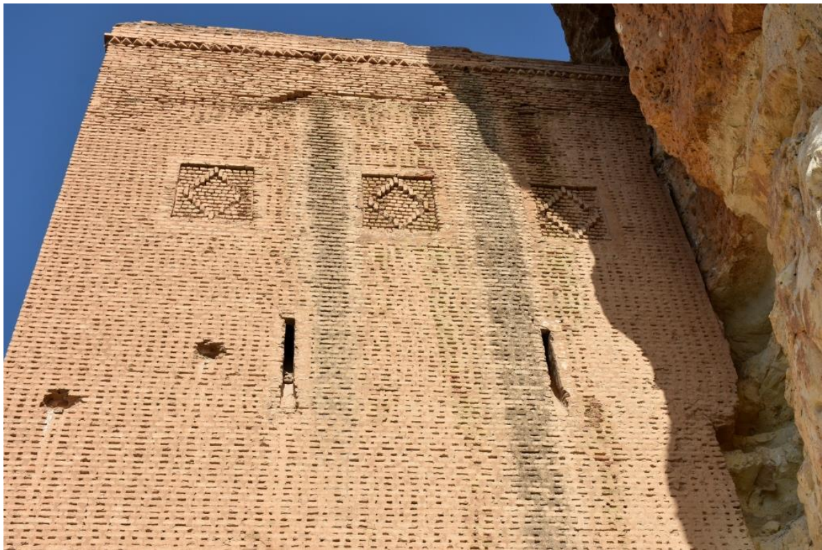
Aliaa Tower (T30) hit by light and medium weapons, Photograph: Zardasht Ezzo, February 2021
