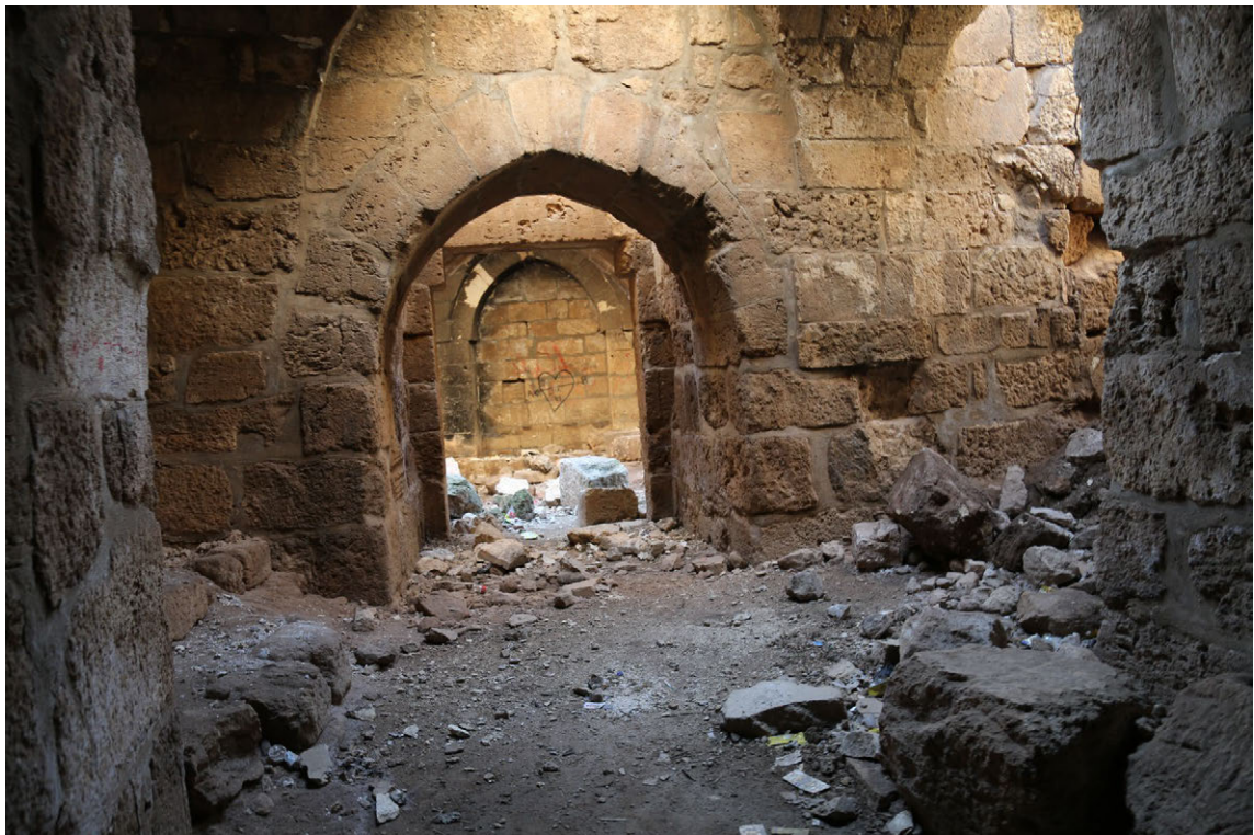
The collapse in the ceilings inside the inner passages ( Damage J ).
