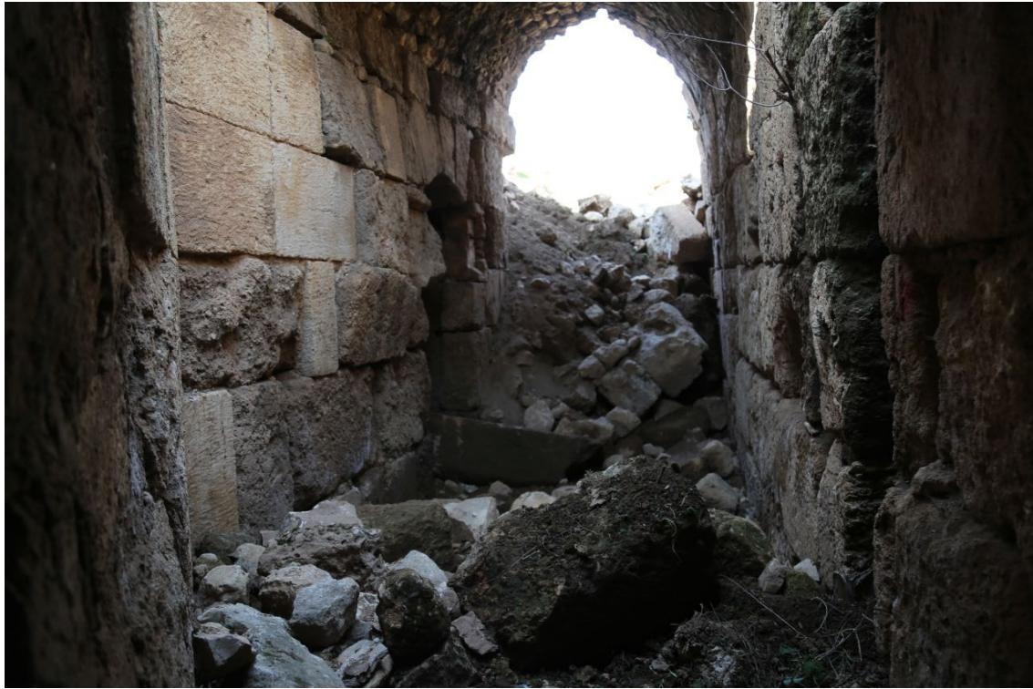
The collapse in the ceilings inside the inner passages ( Damage H ).
