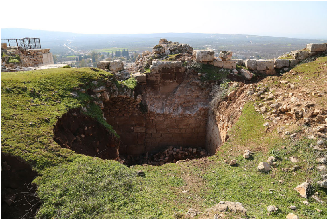
The collapse of the ceiling of the soldier's area ( Damage E )
