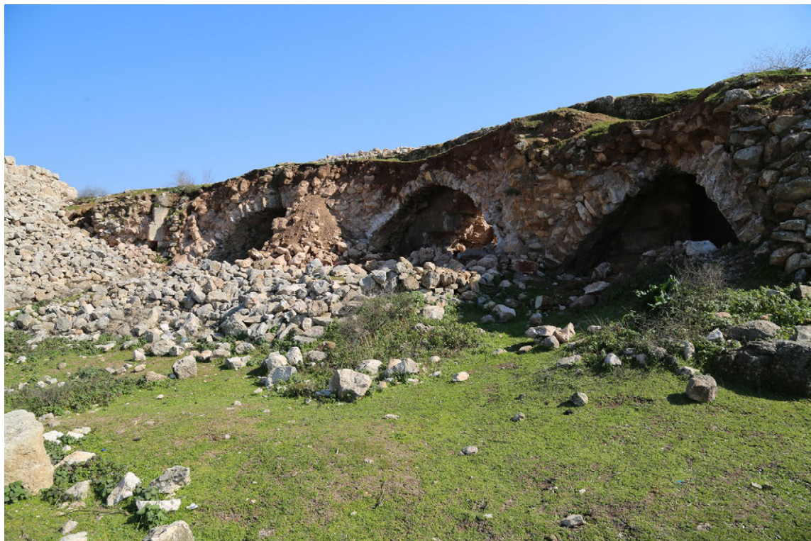
The collapse of the facades of the storerooms ( Damage C )
