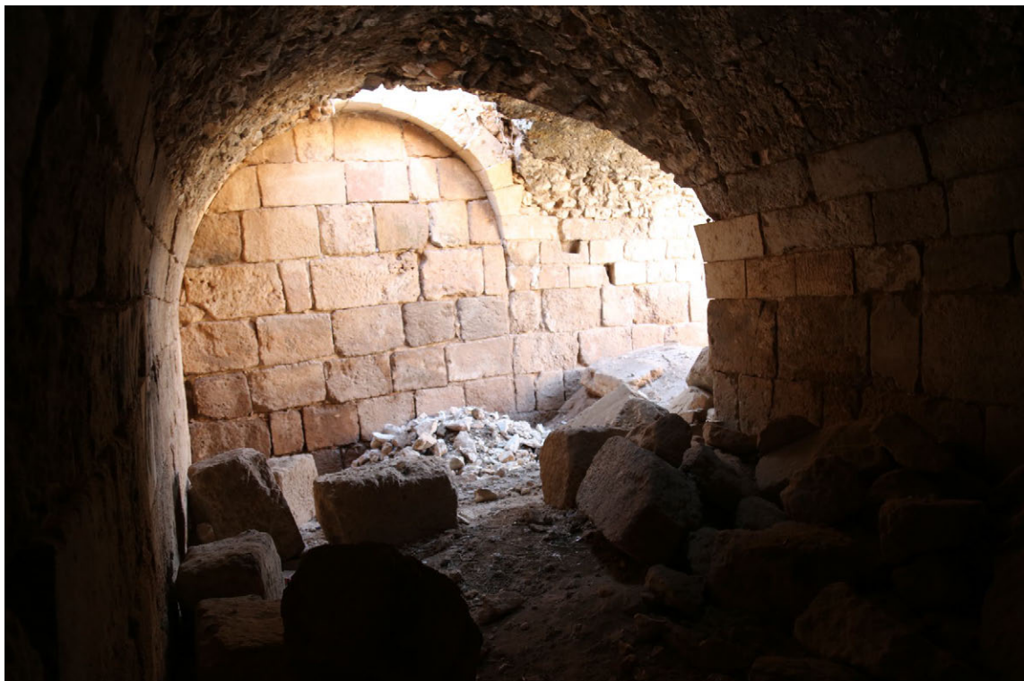
The collapse in the ceilings inside the inner passages ( Damage H ).
