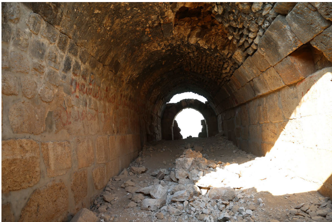
The collapse of some roofs and internal walls ( Damage K )
