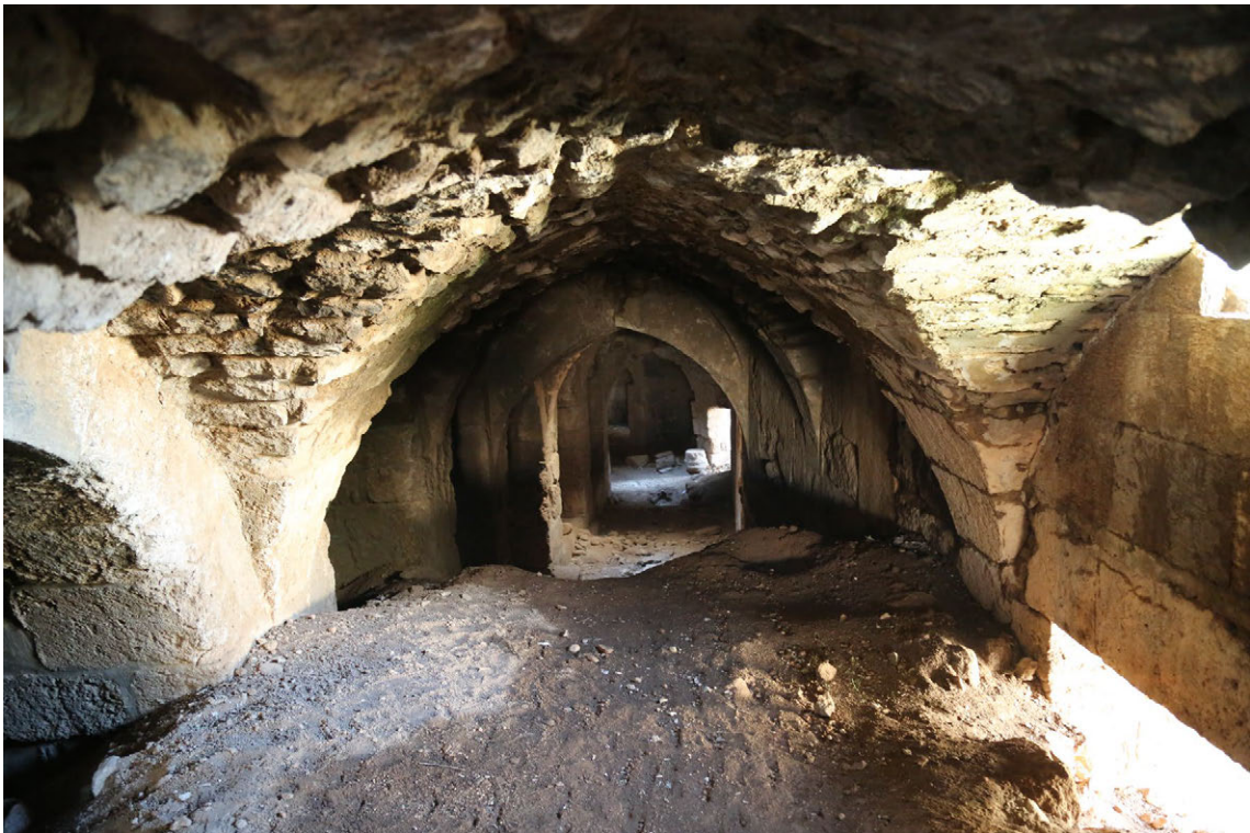
The collapse in the ceilings inside the inner passages ( Damage I ).
