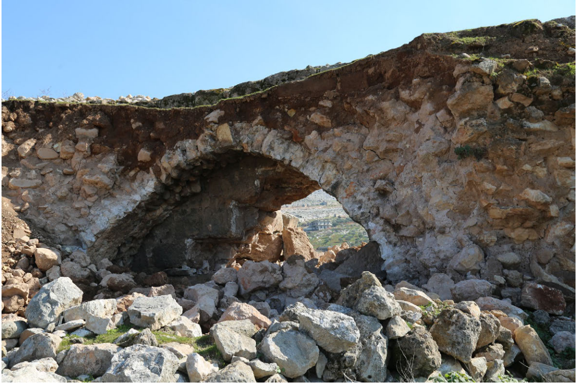
The collapse of the facades of the stores ( Damage D )
